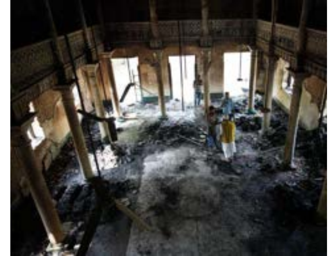
Ukraine: The destroyed library in Chernihiv. Photo – UNIAN.
