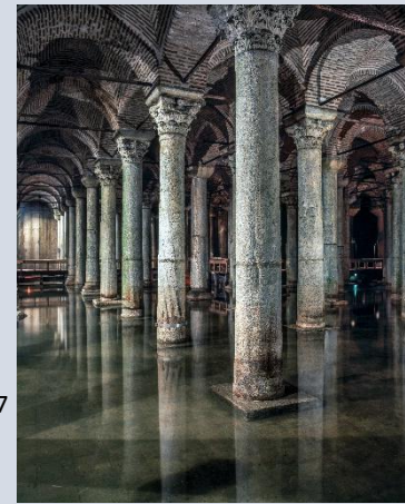
Basilica Cistern, İstanbul, 1997, Aydoğmuş, Tahsin, baz004
